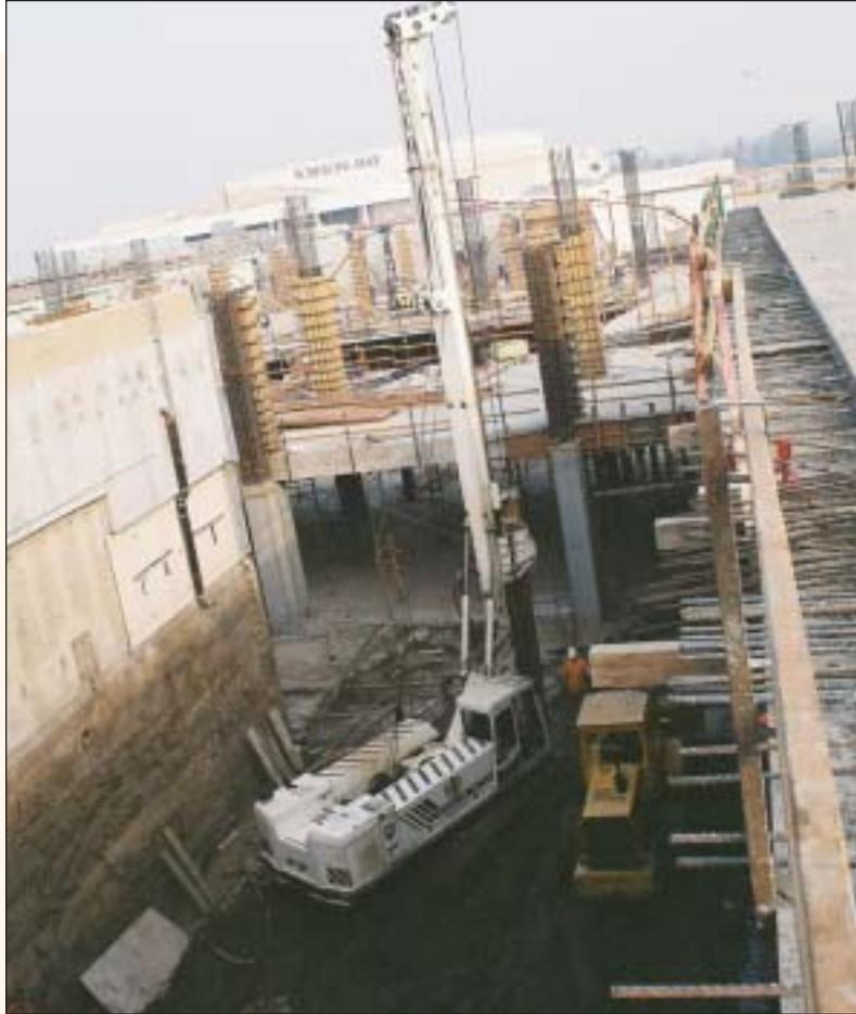
*Into this confined area, Magco stuffed our Mait 130 drill rig, Cat 930 loader 75' long tremie and 60 ton Grove Rough Terrain crane.*
