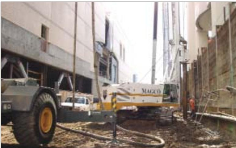
*Installing 1,331 Drilled shaft foundations at Westfield Shopping Town Parking Structure Canoga Park, Ca. Magco Drilling's largest drilled shaft project to date.*
